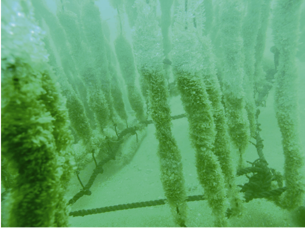
图3 2006年在茂名海底管线路由区铺设的人工海草 Fig. 3 In 2006 artificial seaweeds were fixed to hanging segments of submarine oil pipelines in Maoming
